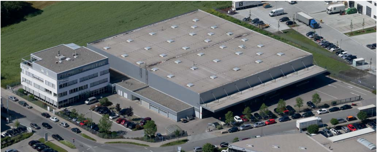
MayTec GmbH plant in Dachau
