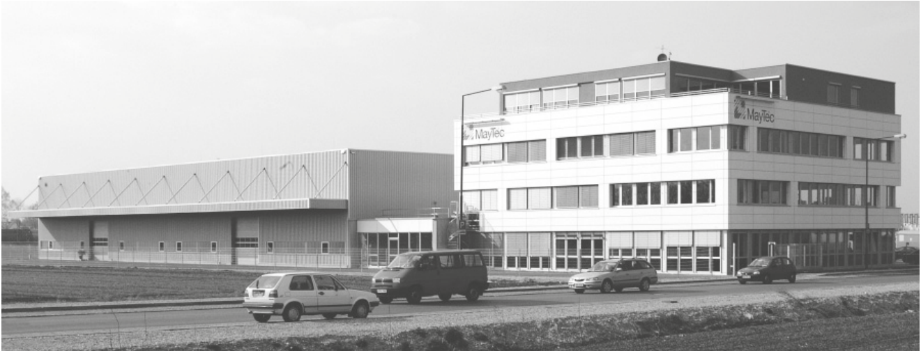
MayTec GmbH plant in Dachau
